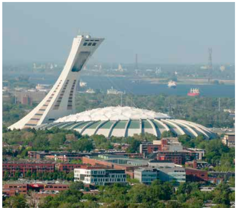
Completed stadium with tower and retractable roof
